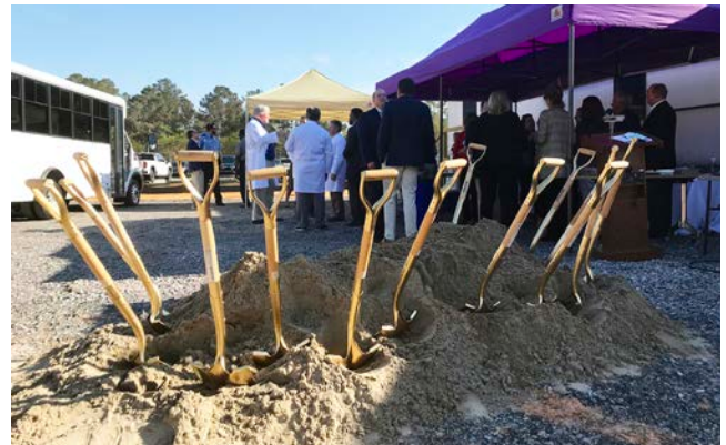
Members of the St. Tammany Health System Board of Commissioners and other dignitaries gathered Nov. 2 to break ground on the health system's new surgery center. The 126,000-square-foot building, which will boast 12 surgical suites, is expected to be ready for patients by late summer 2024.
